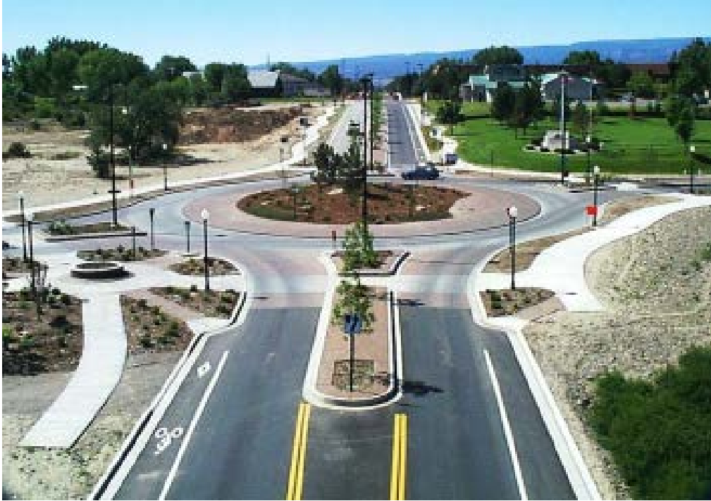
Figure 3.55– Example Pedestrian and Cyclist Treatment (Source: NCHRP 672 2 )
