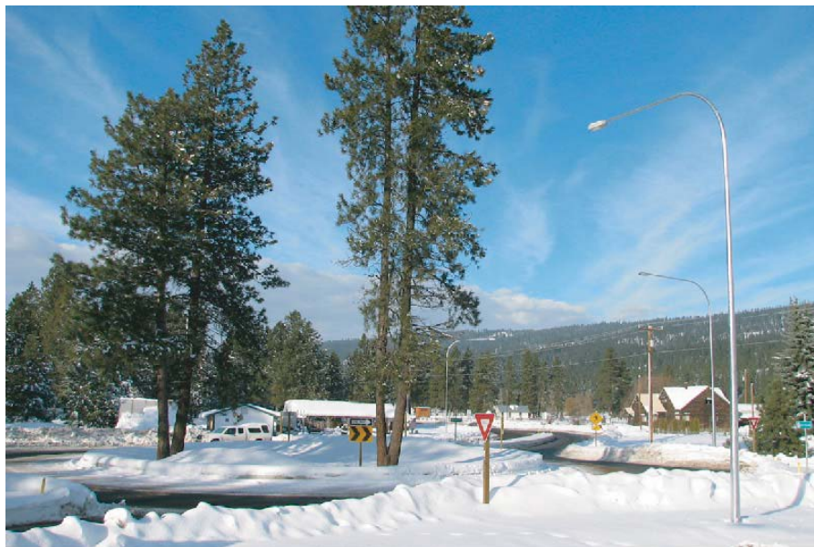
Figure 8.2 – Typical Snow Removal Activity around a Roundabout (Source: NCHRP 672 1 )
